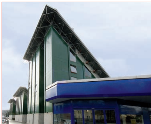
St. Gallerstrasse 106 (green towers)
